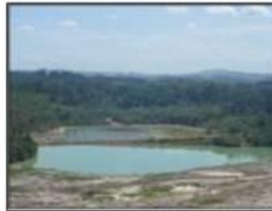
Check Dam (F4Timur)
