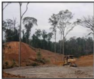
Pembersihan Lahan Bulldozer, Excavator, Chainsaw
